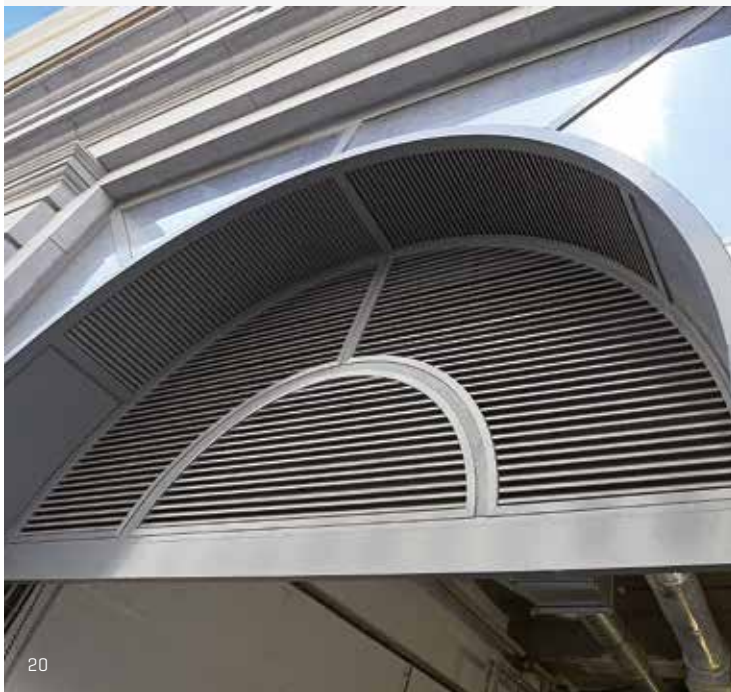
421 - Wall louvre, heavy-duty series
