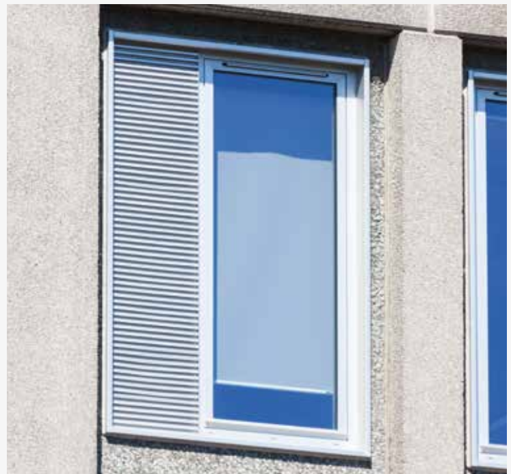
431 - Surface-mounted wall louvre
